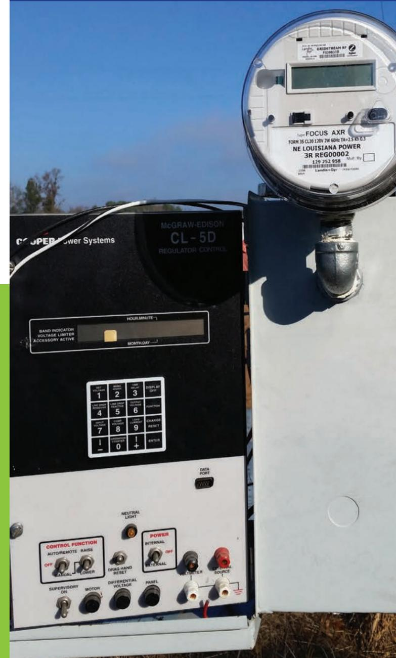
Gerald Hilbun remembers a time when voltage regulators came from the factory with a meter socket for attaching a thermal meter. That recollection provided inspiration for a project using advanced residential meters as sensors to monitor line regulators.
